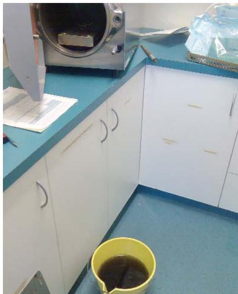
*Figure 1. The water in the bucket has just been drained from the reservoir of the steriliser above and shows severe recycling contamination. The water in this steriliser had not been changed in six months. This is a common sight for technicians servicing sterilisers in busy practices.*
